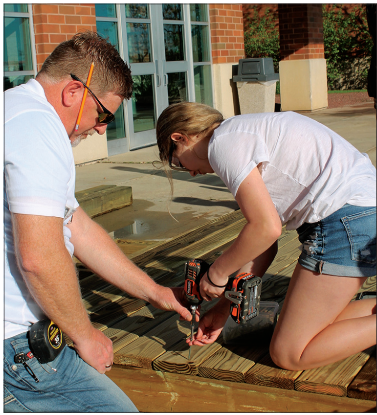
Above: Hoekstra secures a board to the base of the playhouse with an electric screwdriver. At left: After measuring where to cut, Suttman operates the saw under close supervision from Ingersoll.
